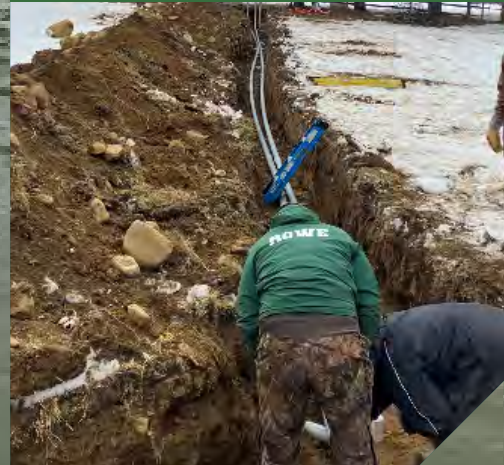
Electrical contractors restoring service cottages at Campo Plymouth State Park.
